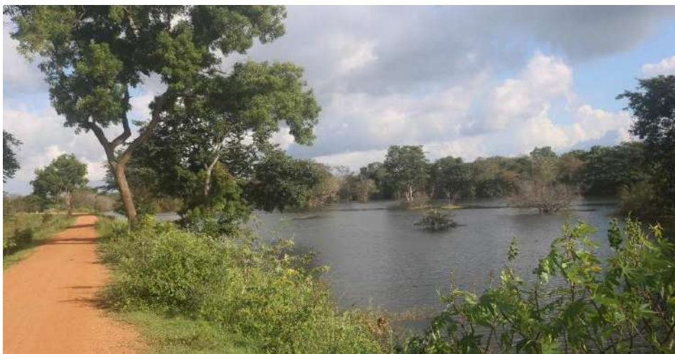
Figure 5: Site view of Thumbikulama Tank after restoration (2024)
