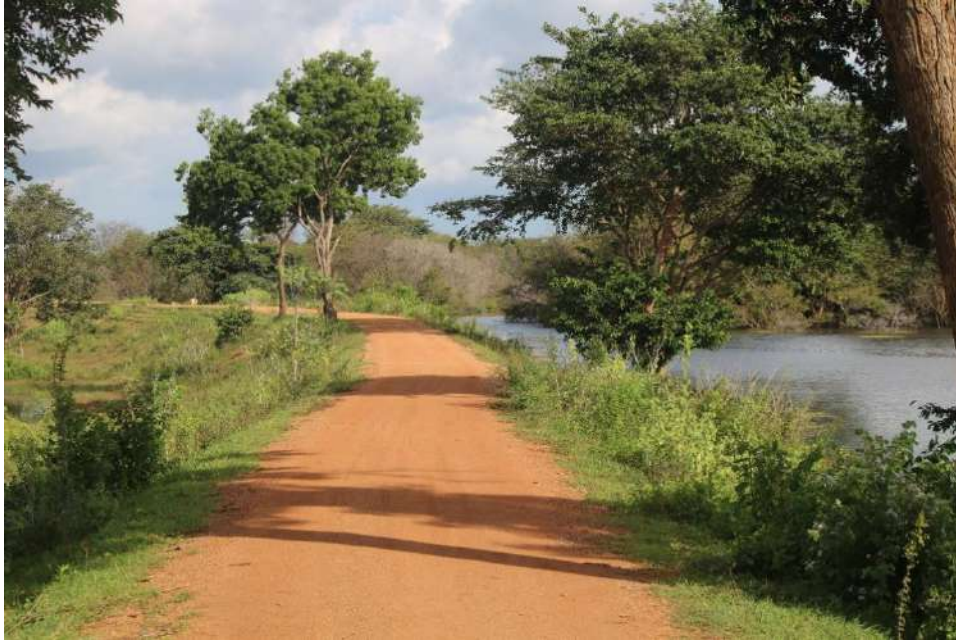
Figure 8: Repaired bund of Thumbikulama Tank
